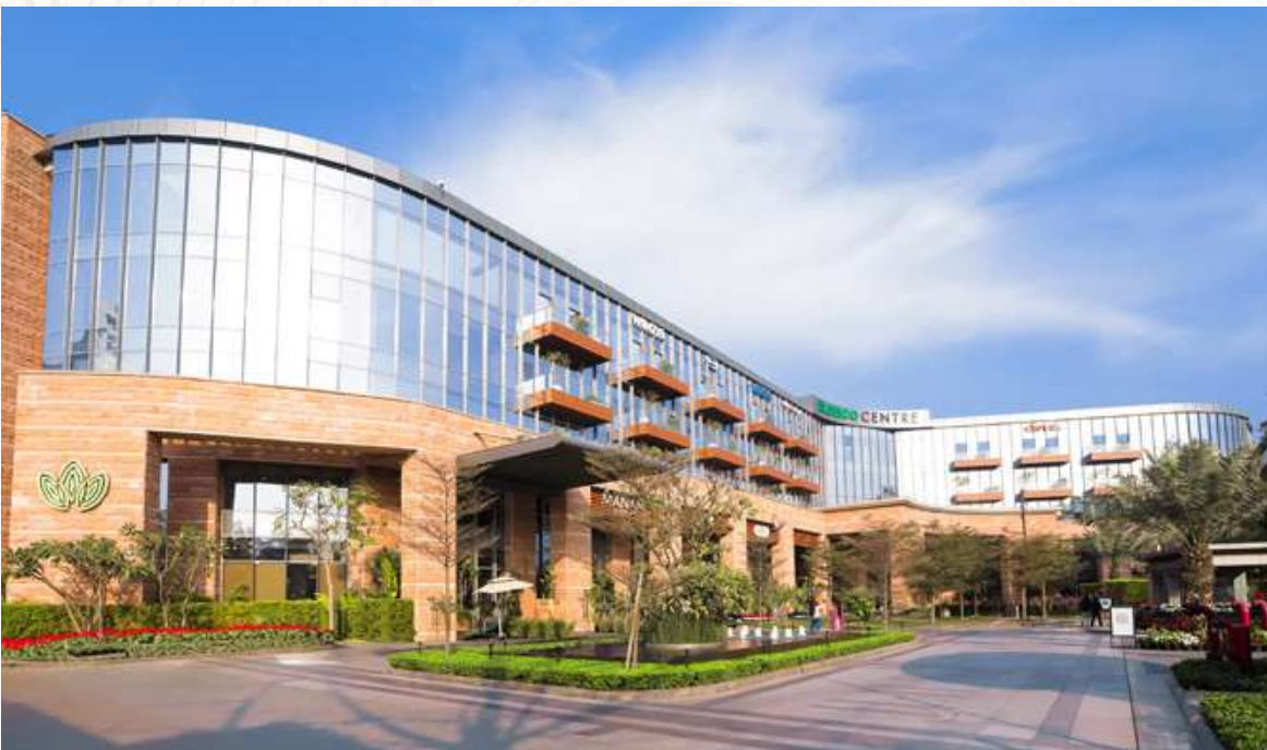
Eldeco Centre (New Delhi) Designed by DFI
